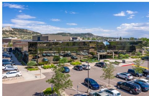
NORTH CREEK 5725, 5755, 5775 Mark Dabling Blvd 980-11,427 RSF Renovated Common Area, Fitness Center, Training/Conference Center
