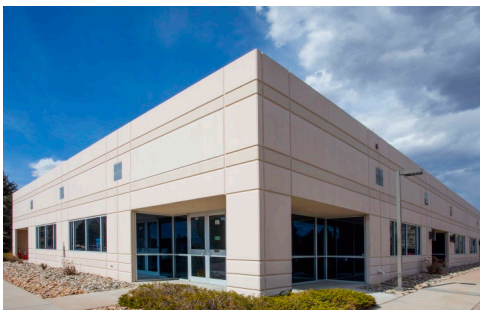
CENTENNIAL TECHNOLOGY CENTER 4920 Centennial Blvd 59,970 RSF For Sale of Lease
