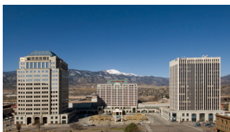
Palmer Center 2 N & 90 S Cascade Ave 924 to 8,403 SF For Lease
