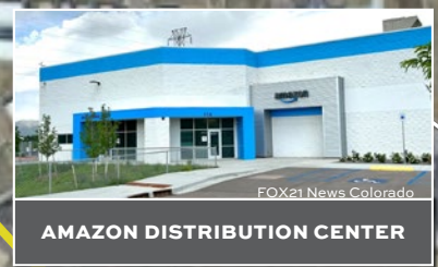
AMAZON DISTRIBUTION CENTER
