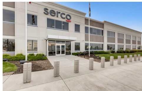
1055 NEWPORT 1055 N Newport Road 5,292-31,190 RSF New ownership, Class A office, SCIF
